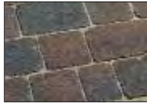
PARKING BAYS MARSHALLS TEGULAR CONCRETE PAVING COLOUR BURNT OCHRE
