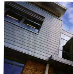
HORIZONTAL METAL PLANKS ECHOING THE FEEL OF WEATHER BOARDING
