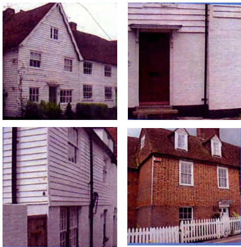
PUB ELEVATIONS (BELOW) DESIGNED TO HAVE A KENT CHARACTER WITH WEATHERBOARDING, RED BRICK, TILED ROOF, GLAZING BAR PATTERN AS SHOWN IN THE EXAMPLES ABOVE
